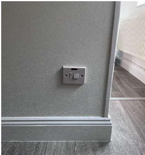
Figure 3- Hot water heater isolator switch and Heater On / Off switch location
