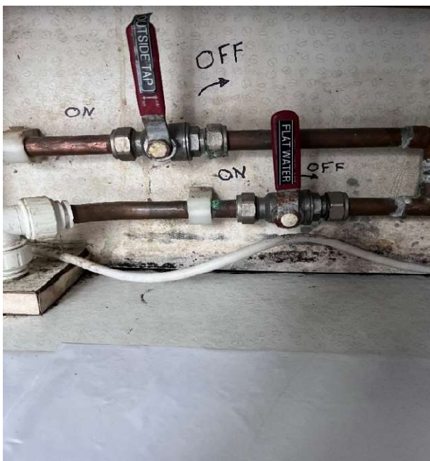
Figure 4- Cold water isolator valves
